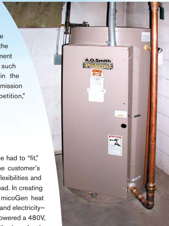
*The Capstone MicroTurbine's electrical output drives this additional water heater.*
