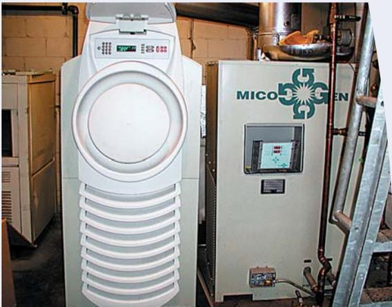
Clean exhaust heat generated by the Capstone MicroTurbine loops into the Holiday Inn's commercial grade boiler via a heat exchanger.
