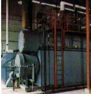
The Donlee TurboFire™ XL boiler, installed at Knouse Foods, reaches production capacity of 34,500 pounds of steam per hour (at 125 psi) within 30 to 45 minutes of start-up.
