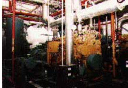
*The Omstead Foods plant employs two natural gas-fueled Caterpillar engines to drive ammonia compressors for freezing and refrigeration. Both engines are direct-drive to the compressors, eliminating the cost and maintenance of gear costs.*
